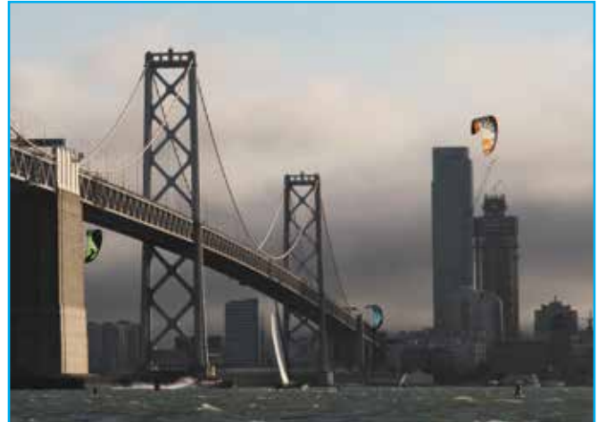
Redevelopment of the Island and open space in this area was designed to enhance boardsailing access at this iconic location, but delays have made its proper implementation questionable. Future redevelopment should incorporate access to the area's world-class winds (Photo: Erin Loscocco).
