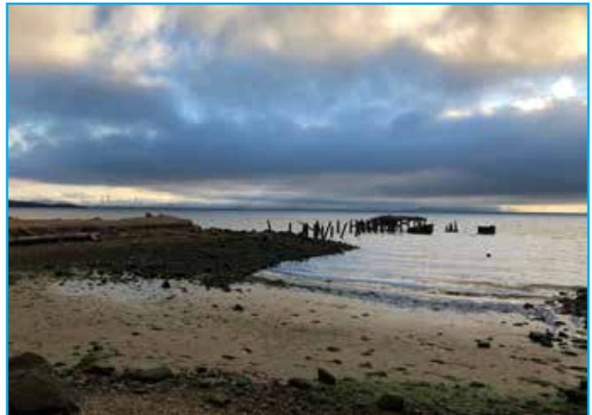
Hazards to kiteboarders are located on three sides of the beaches, including riprap shoreline and old pier pilings. These hazards, combined with the need to immediately get upwind, makes Fleming Point suitable only to advanced kites (Photo: Andrew Sullivan).
